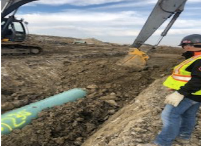
Excavator backfilling tie-in– km 152+640– Oct 18, 2018
