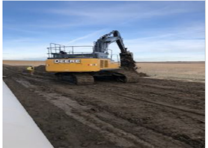
Excavator digging ditch for mainline crew – SF 103 – Oct 15, 2018
