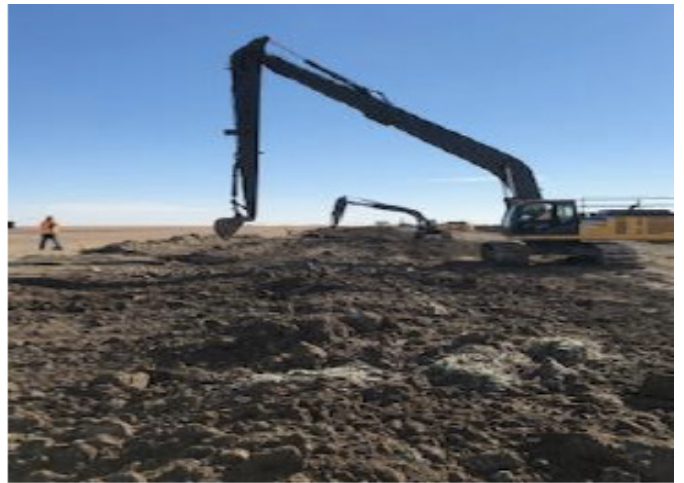
Main line backfill crew pulling soil – km 185+100 – Oct 20, 2018
