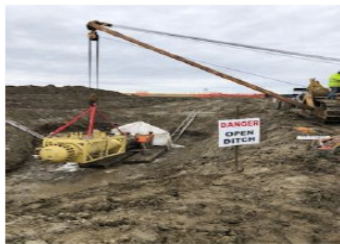
Welding on pig catcher – km 178+300 – Oct 15, 2018
