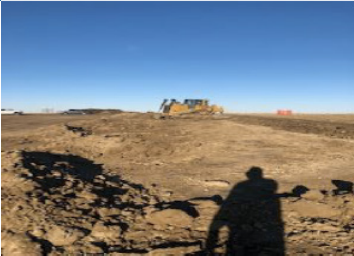
Dozer grading on Native Prairie – km 254+178 – Oct 17, 2018
