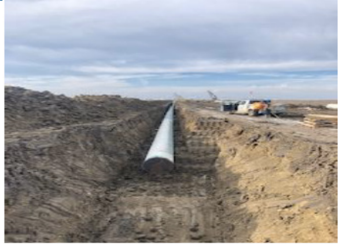
Mainline lowered into ditch– km 181+900 – Oct 18, 2018
