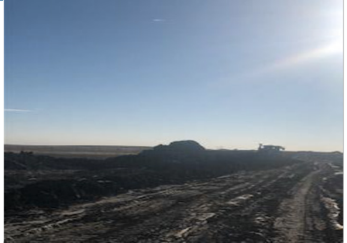
Dozer pushing clay into tie-in backfill – km 151+800 – Oct 20, 2018
