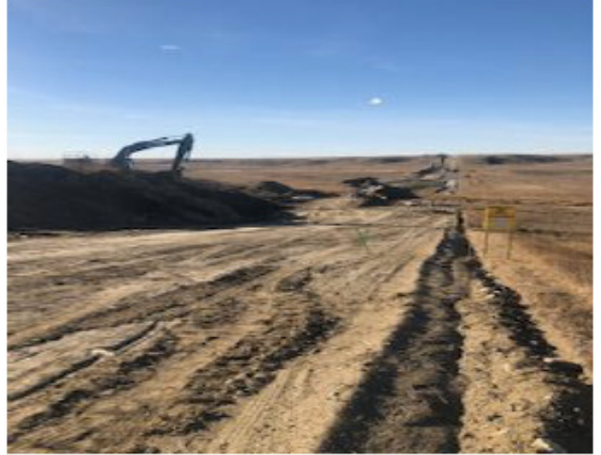
Excavator moving spill pile – km 255+180 – Oct 19, 2018
