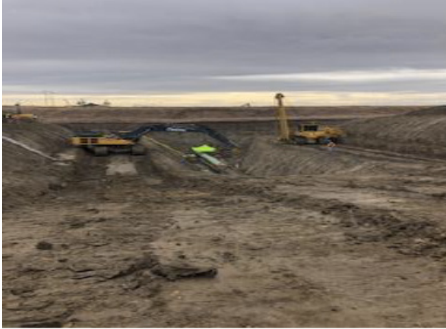
Track bore crew – km 193+300 – Oct 15, 2018
