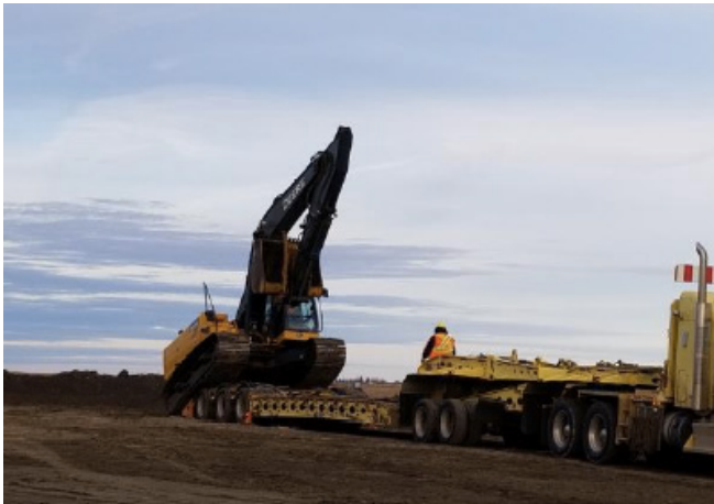
Loading equipment – km 266+700 – Oct 15, 2018
