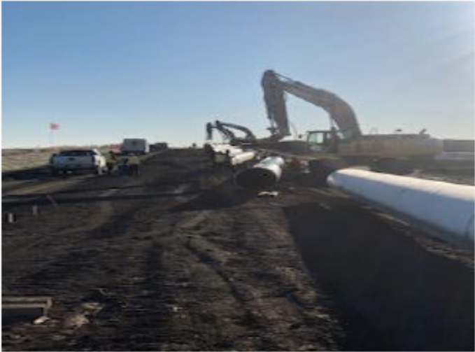
End prep crew - km 214+700 – Oct 19, 2018
