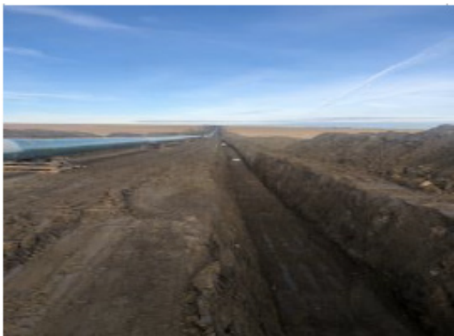
Ditched mainline – km 172 to 173 – Oct 15, 2018
