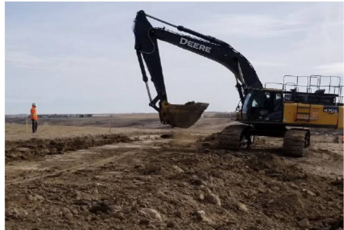
Grading sensitive area with Archaeologist onsite – km 254+300 – Oct 15, 2018
