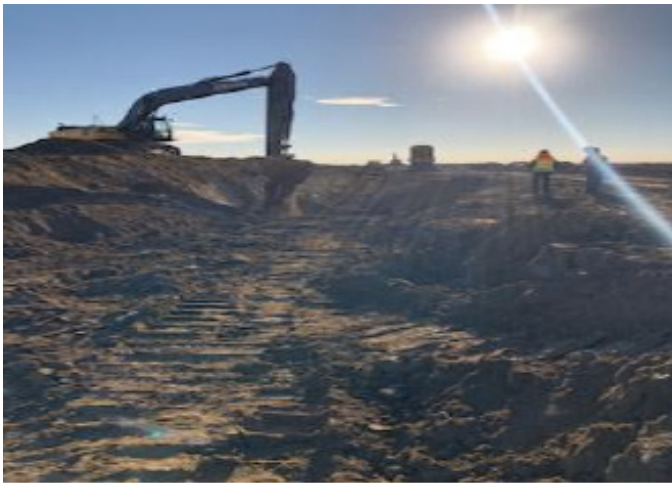
Backfill and shading bell holle - km 151+840 – Oct 20, 2018
